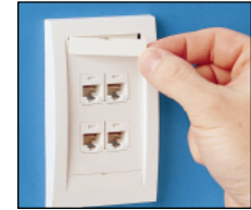
3. Snap screw cover onto faceplate
