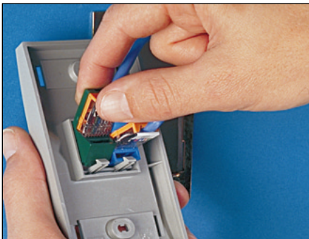
1. Snap in terminated MINI-COM modules.
