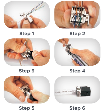
SL Series Modular Jack Termination Tool UTP Termination Method
